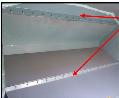
**The bin dividers must be fully sealed with silicon** as air leaks internally between the bins can be detrimental to the accuracy of the sowing operation. Refer [Page 5.1](#)
